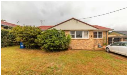
181 Ballina Road, Alstonville
