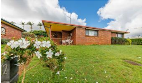
12 Arrowsmith Avenue, Alstonville
