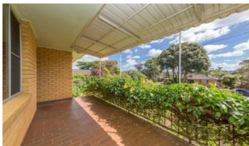
2 Suncrest Avenue, Alstonville
